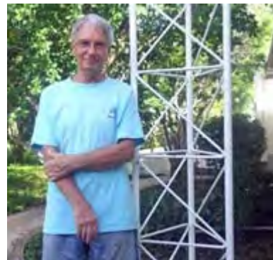
Base of the 80 foot "US/JA" tower with epoxy paint to protect against corrosive sea air.
