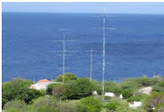
Antennas at PJ2T include stacked monobanders on 10 meters, long-boom monoband Yagis on 15 and 20 meters, and a 40 meter Yagi. [Photos by permission of Geoff W0CG, PJ2T.]
